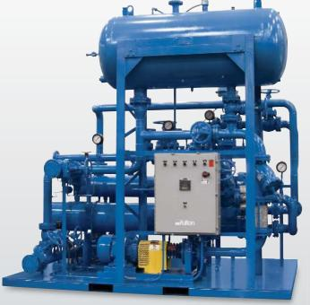
Water is used as the single fluid media for the TCU pictured above, providing heating and cooling for rubber processing. Operating temperatures are between +40°F and +400°F for this highly cyclical application.
